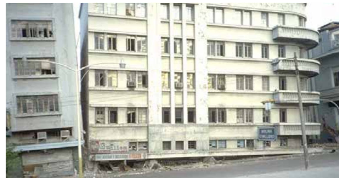
Figura 135. Daños observados durante el sismo de 1986, M5.7 – San Salvador 61 Fuente: Olson, Robert A. Collection. Earthquake Engineering Online Archive, National Information Service for Earthquake Engineering, EERC, University of California, Berkeley
