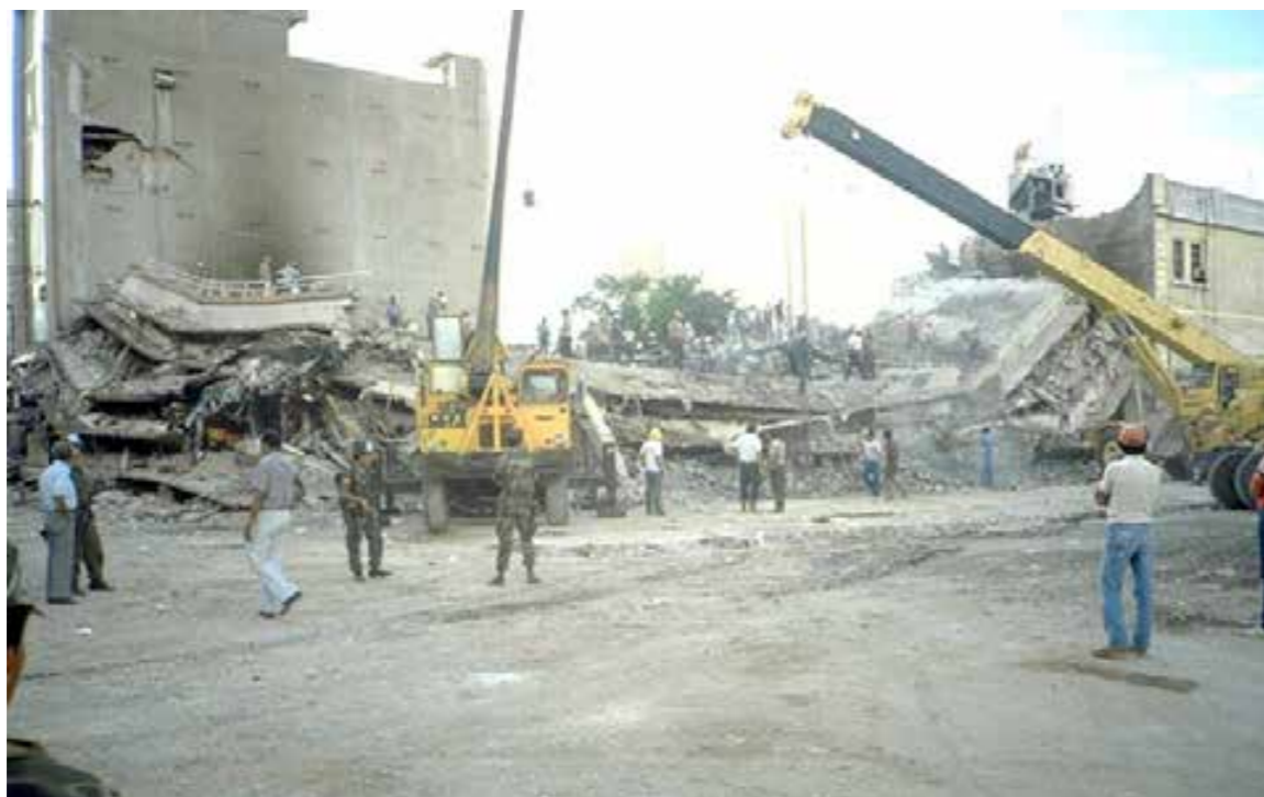
Figura 133. Daños observados durante el sismo de 1986, M5.7 – San Salvador 61 Fuente: Olson, Robert A. Collection. Earthquake Engineering Online Archive, National Information Service for Earthquake Engineering, EERC, University of California, Berkeley
