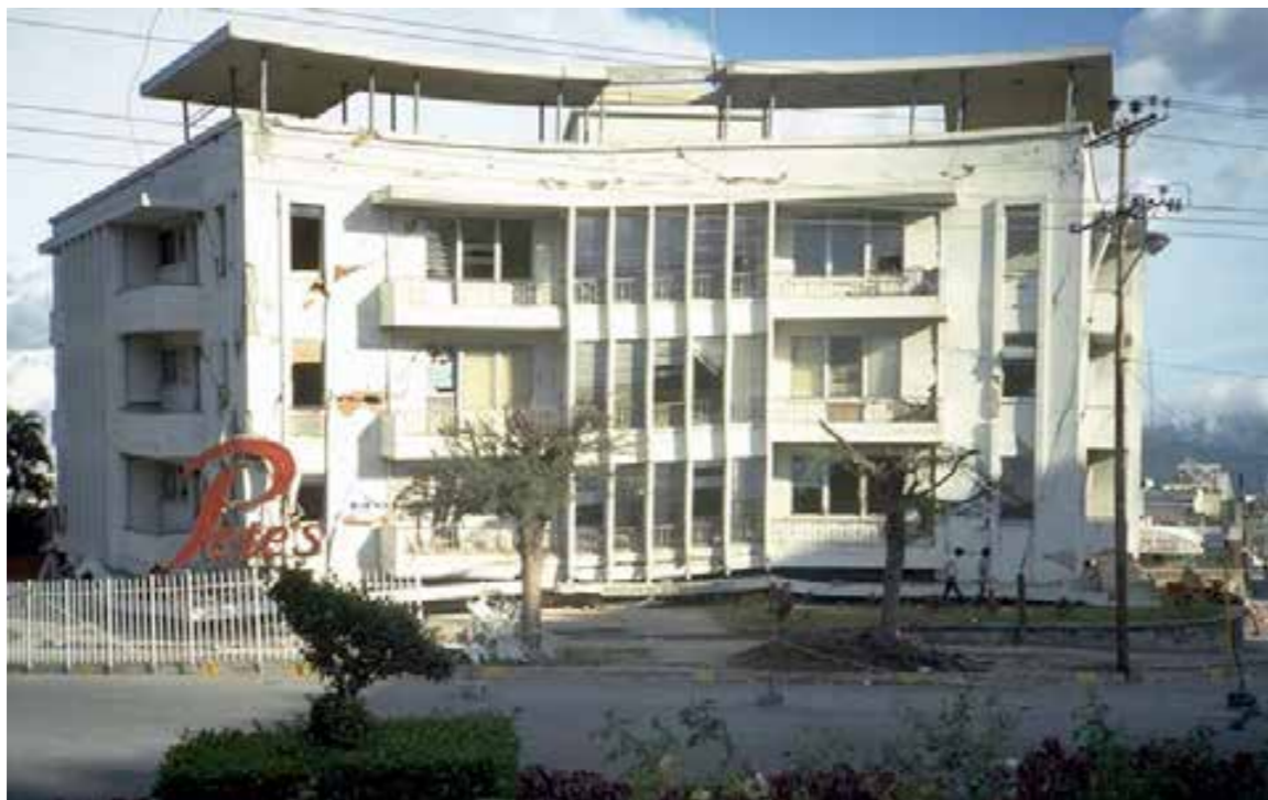
Figura 134. Daños observados durante el sismo de 1986, M5.7 – San Salvador 61 Fuente: Olson, Robert A. Collection. Earthquake Engineering Online Archive, National Information Service for Earthquake Engineering, EERC, University of California, Berkeley
