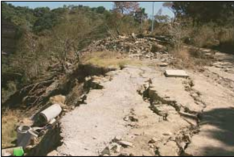
Figure 10. Shattered ridge near Comasagua.
