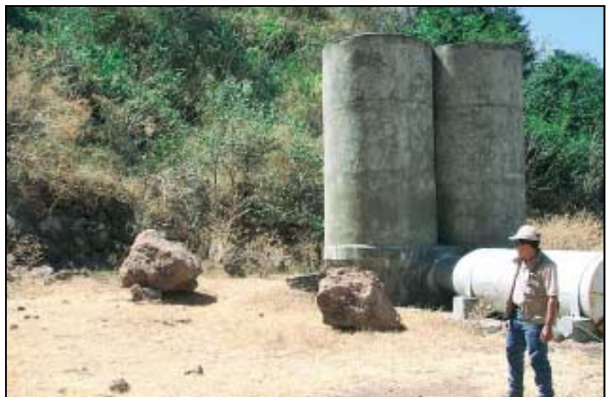
Figure 15. Boulders from rock fall above geothermal well near Berlin.
