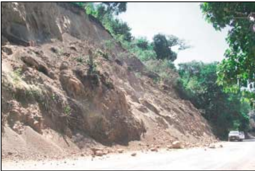
Figure 16. Landslide on road from Berlin to Alegria.
